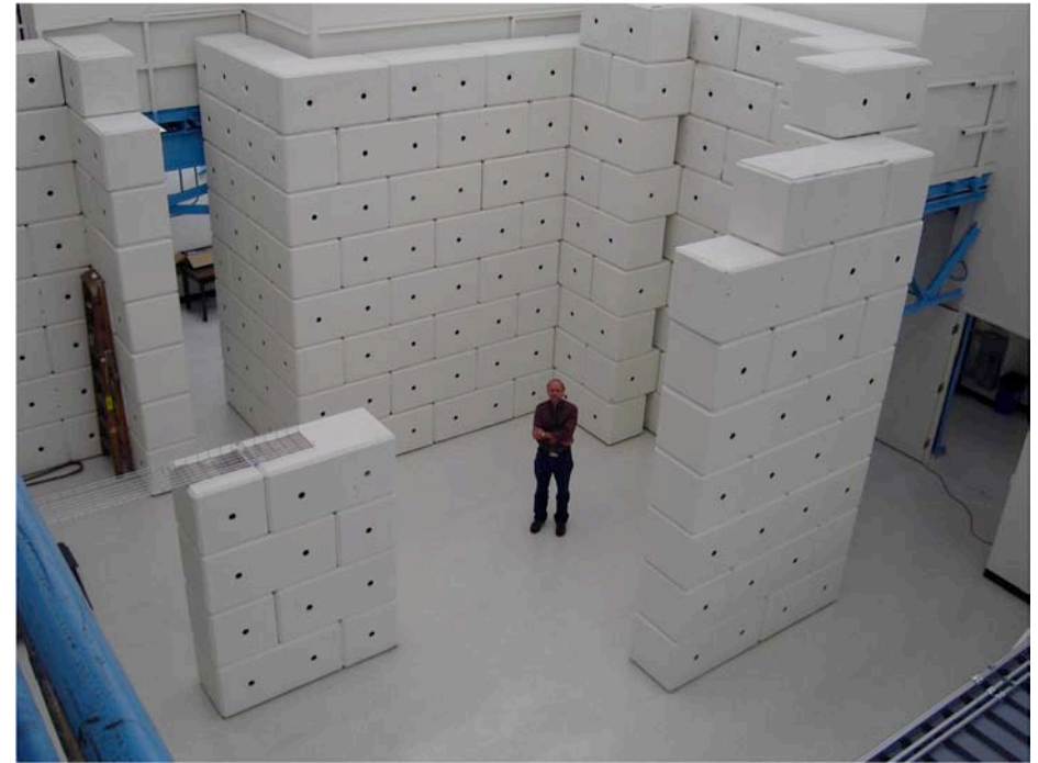
Texas Petawatt Target Bay with shielding installed around the Petawatt beam target area
