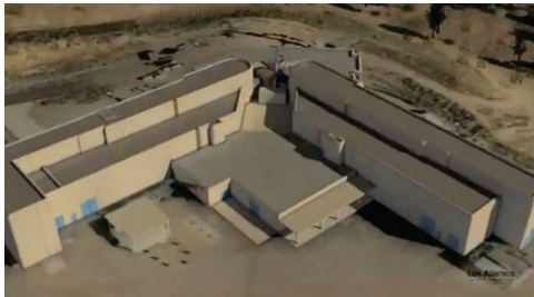
Figure 4: The Dual-Axis Radiographic Hydrotest Facility (DARHT) uses two linear induction electron accelerators to provide dynamic radiographs of imploding systems.
