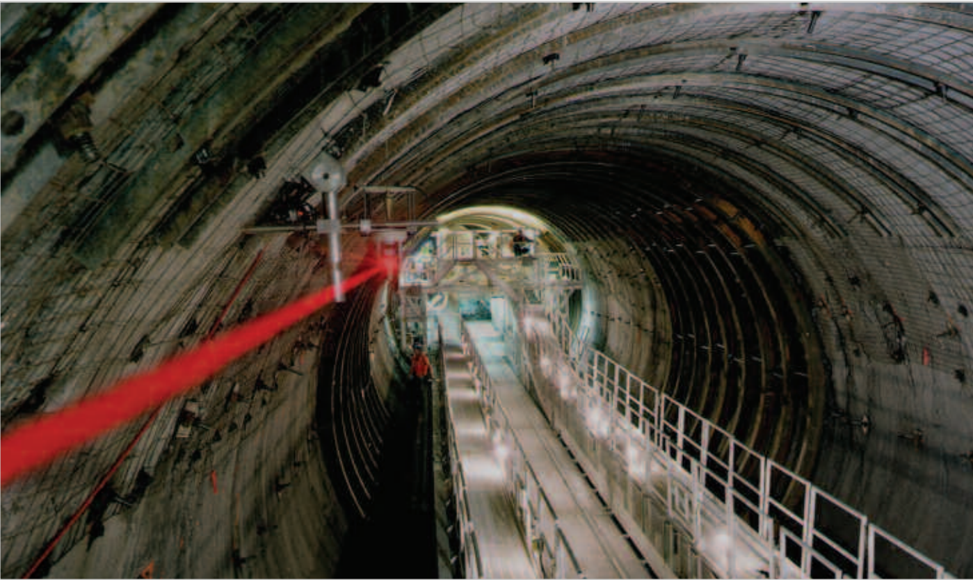
View of the rear of the tunnel boring machine showing the laser guidance system in operation at Yucca Mountain’s Exploratory Studies Facility.
