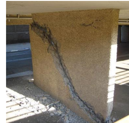
Shear Wall Failure (air-worldwide.com)
