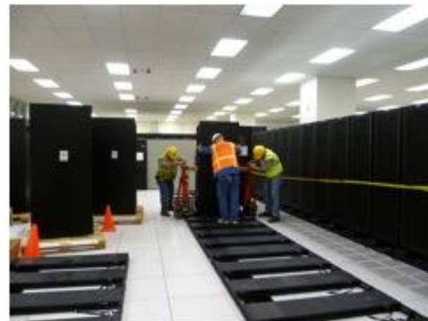
Hopper installation, August 2010
